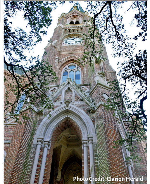
Top: A set of carrara marble Stations of the Cross each over four feet tall and two feet wide depict the passion of Christ inside the church. Bottom: The iconic spire of St. Stephen Church is a steel frame that is wrapped in terracotta tiles. It is 200 feet in height and has 24 sides.
